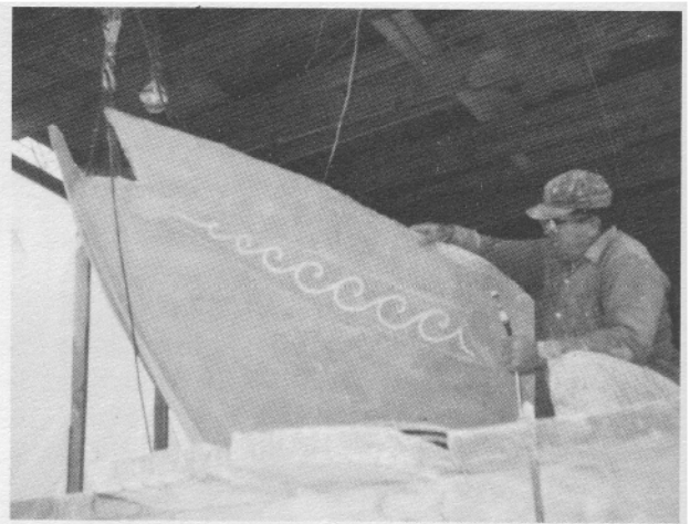
Views of an interesting job being done by Veikko Ackren using FER-A-LITE type mortar to make trailboards for an "Endurance 35".
