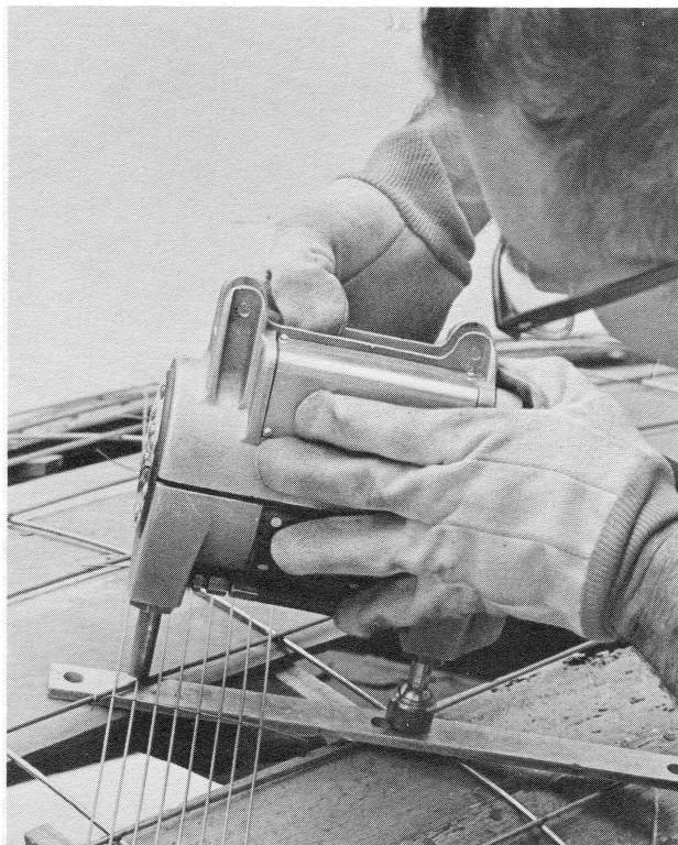
Copper shorting bar is used to increase current at weld. Bar is slipped under edge of last plank applied.
