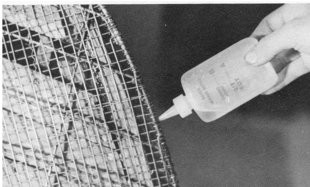
Method used to apply "GIT"-ROT to wrapped joints.
